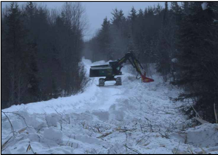
Equipment removing brush on the access road.
