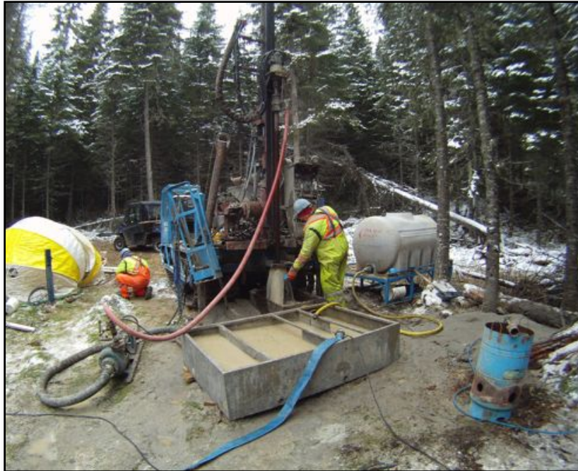
Engineering contractor conducting the pump test in early November 2012.
