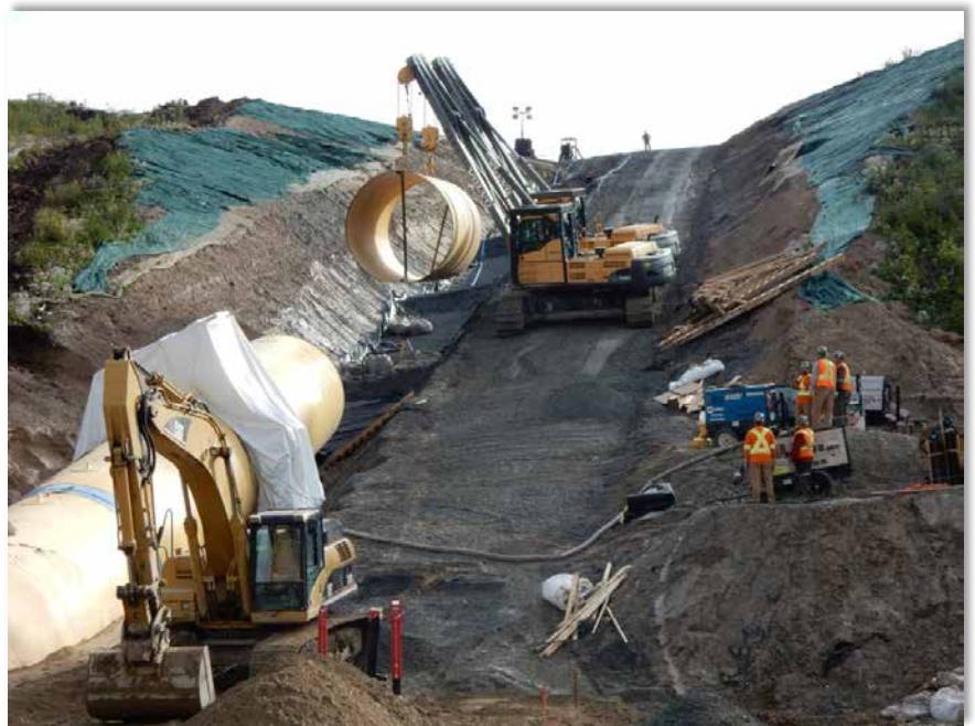
Cranes lower a section of the penstock into position.
