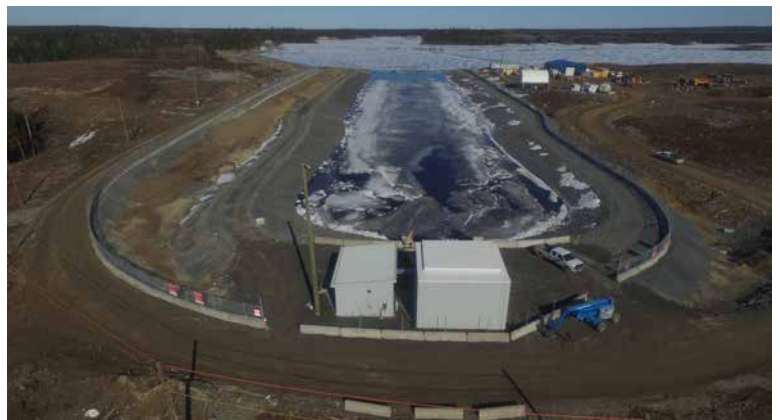
The watered up intake canal.
