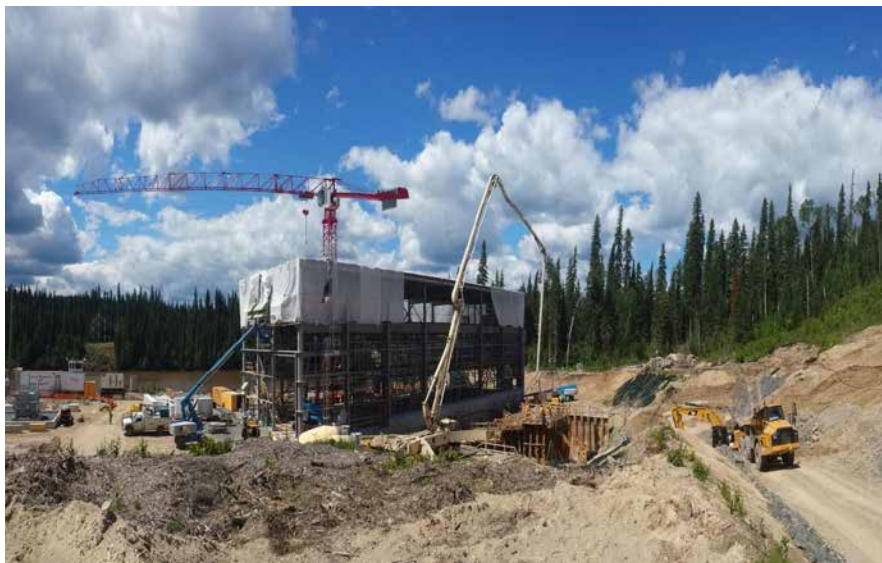
The powerhouse under construction.
